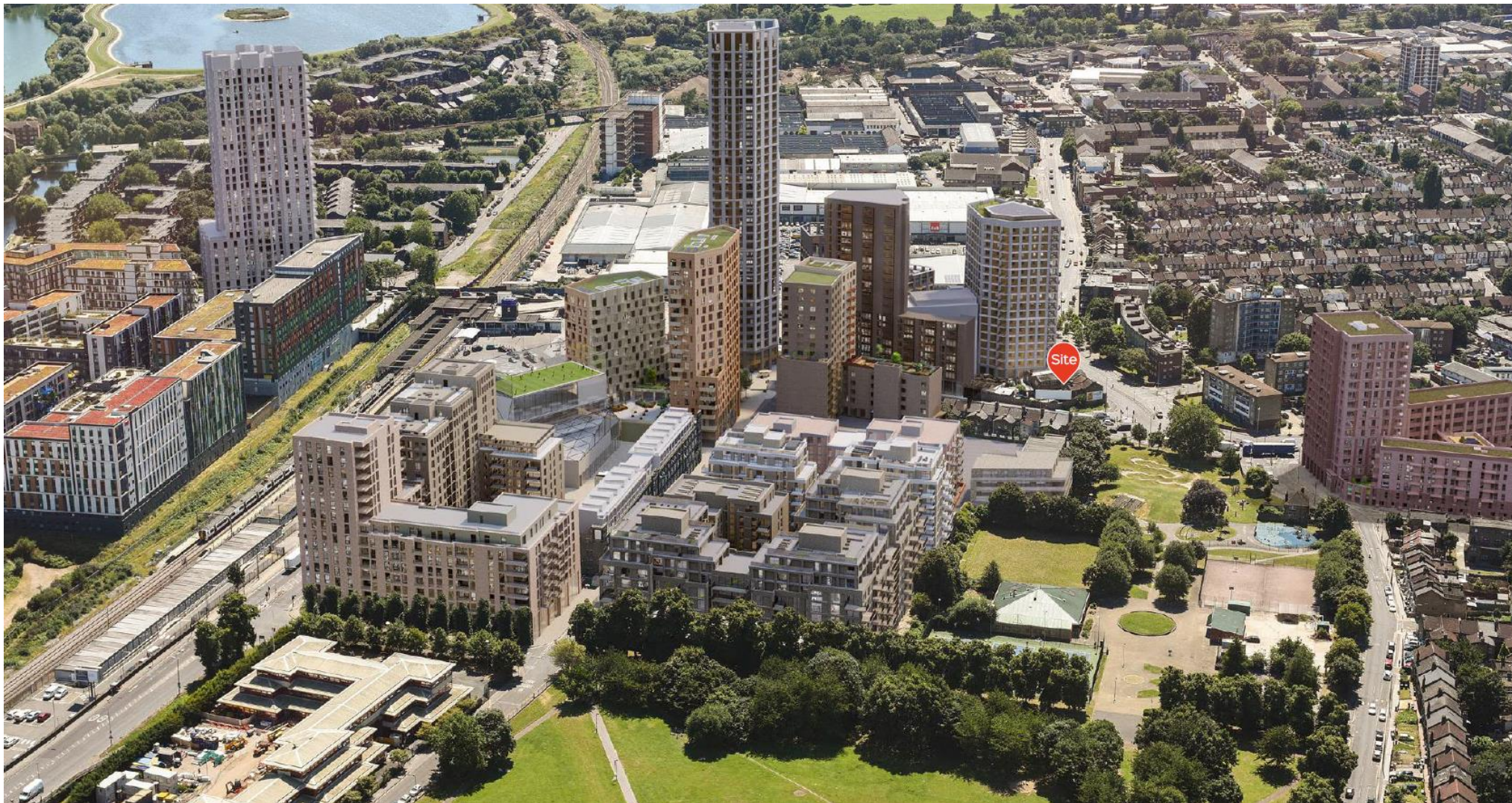
Illustrative view of built out Argent masterplan in the context of other permitted schemes in Tottenham Hale
